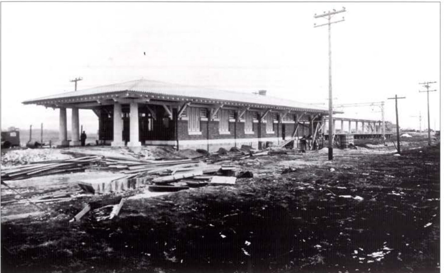
▲ By March 3, 1925, the station building roof has been completed and windows are in place.—Illinois Railway Museum Collection via J. J. Sedelmaier Productions Collection
